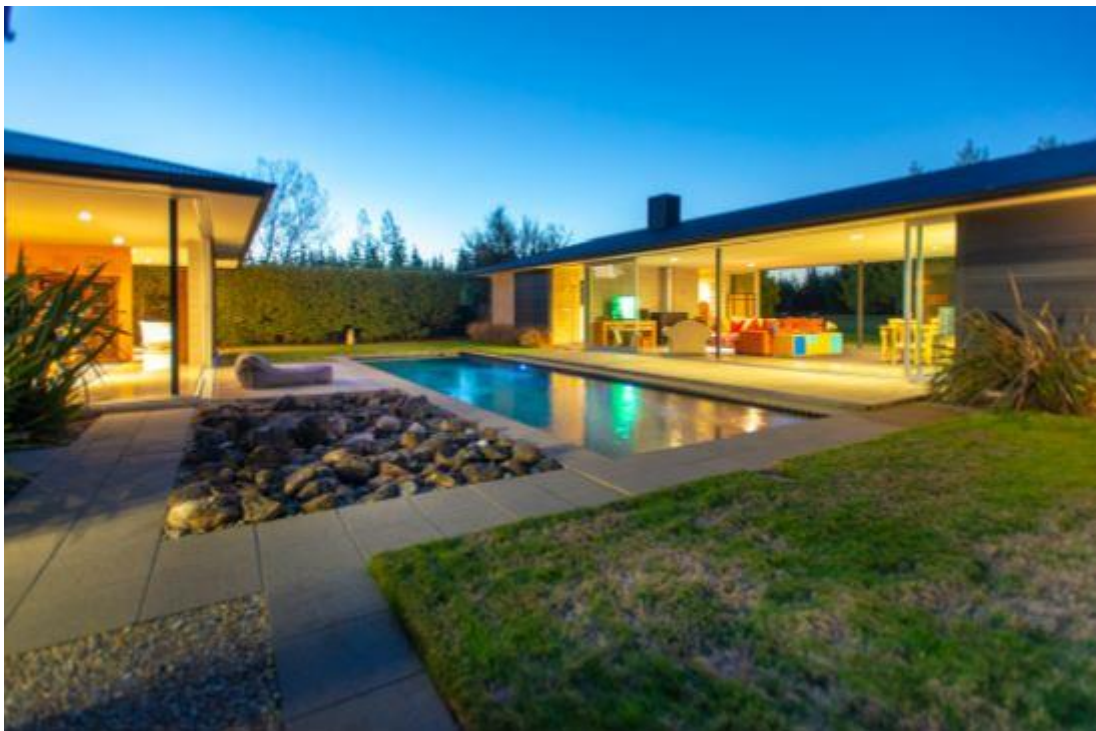
Photograph 1: the house and pool as originally constructed
